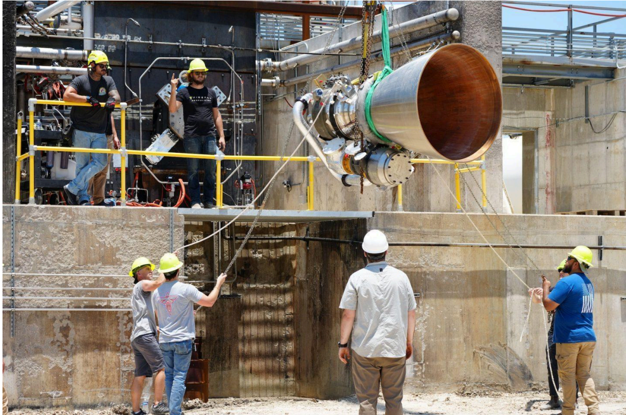
Technicians install a Miranda engine at the test stand in Briggs, Texas. Credit: Firefly Aerospace
